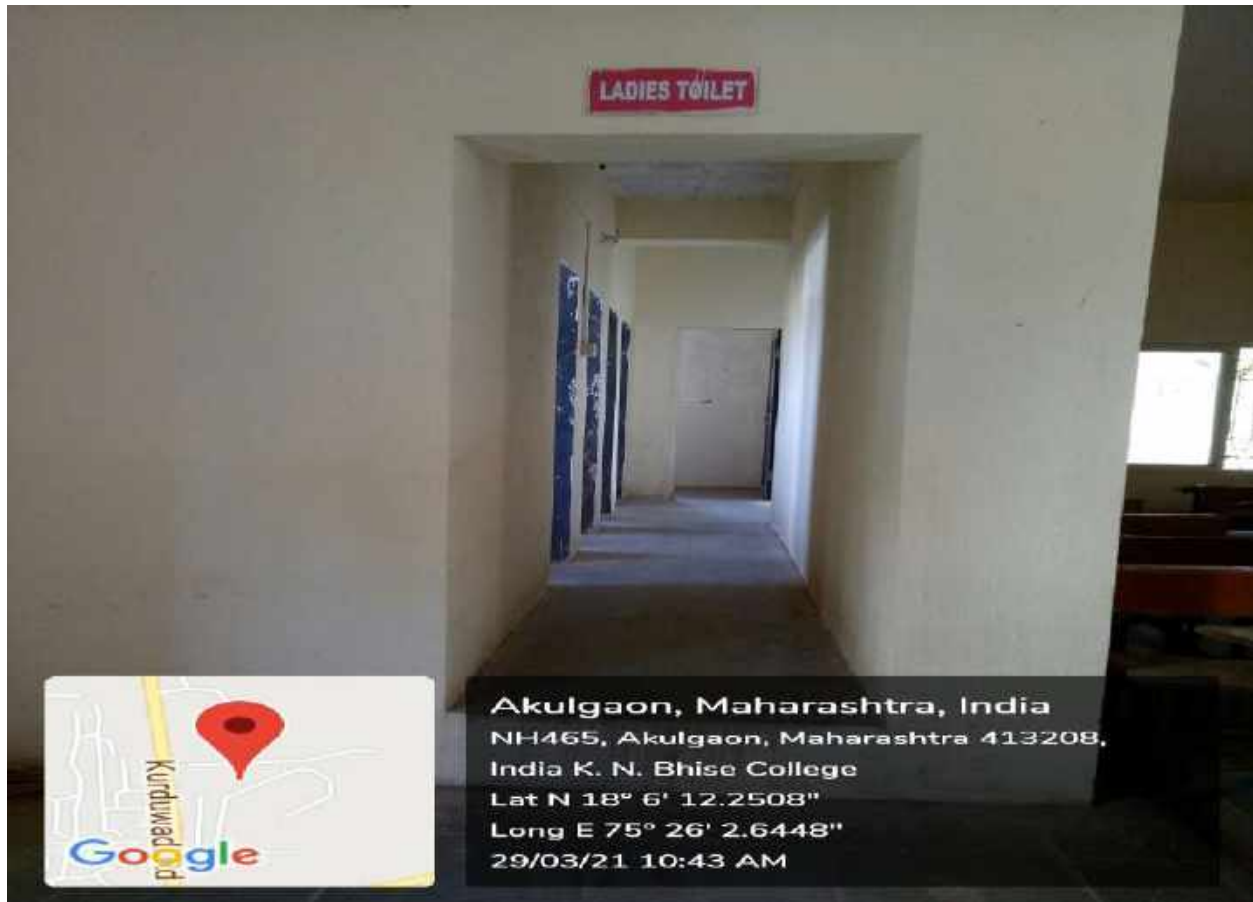
Toilet Facility in Ladies Common Room
