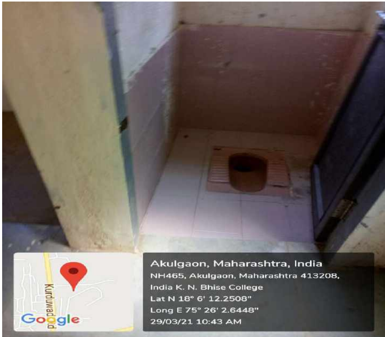
Toilet Facility in Ladies Common Room
